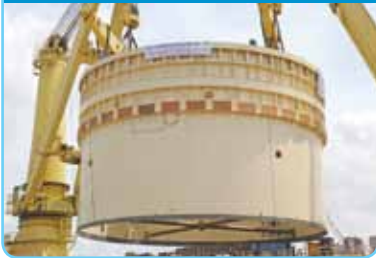
Bogie Support Structure
