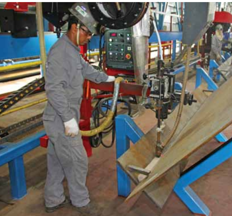
Worker trained to use Semi-Auto Welding Machine (SAW) to improve productivity
