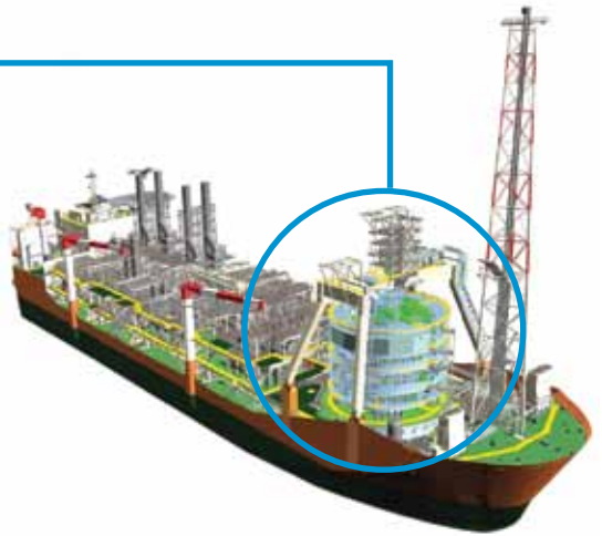
FPSO Glen Lyon
