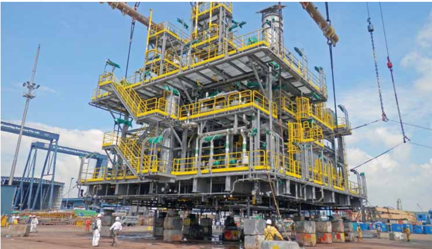
The load-out of FPSO Stones topside modules
